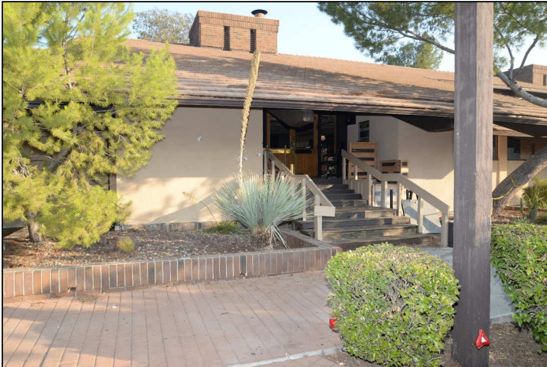
Borderline front stairway and front entrance during daylight hours (the right side door was open during the incident).
